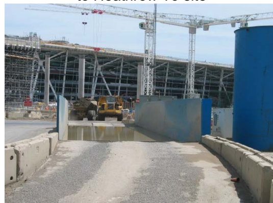
Example: Washing facilities at entrance to Heathrow T5 site
