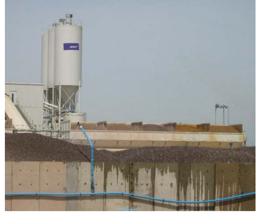
Example: Dust suppression at aggregate store, Heathrow T5
